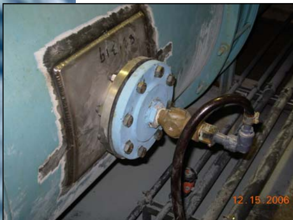
Chemical Feed Pipe After Repair
