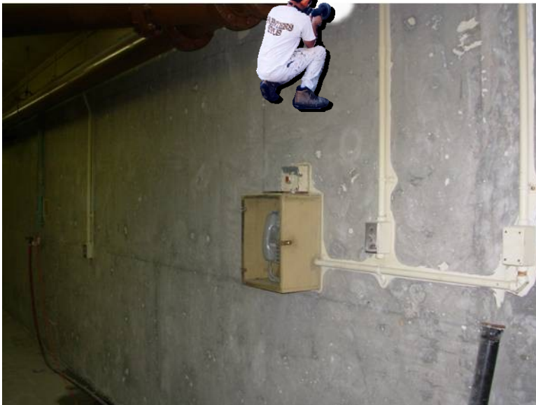
Tunnel surface after several coats of paint have been ground away.
