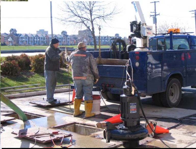
Employees endure harsh weather and a tight working space to install the new parking lot pumps.
