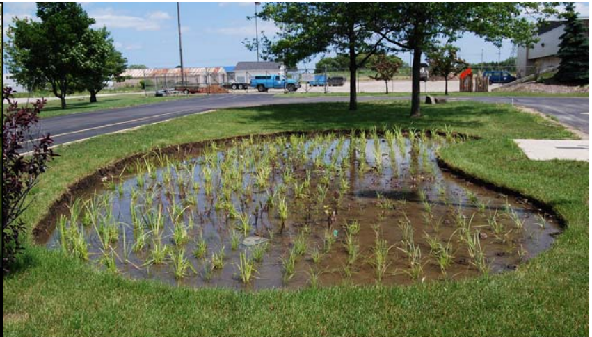
Nearly Completed Rain Garden
