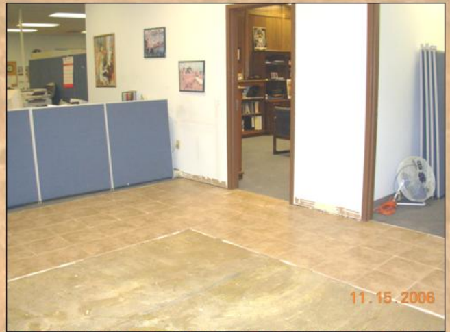
Engineering Reception Area During Renovations
